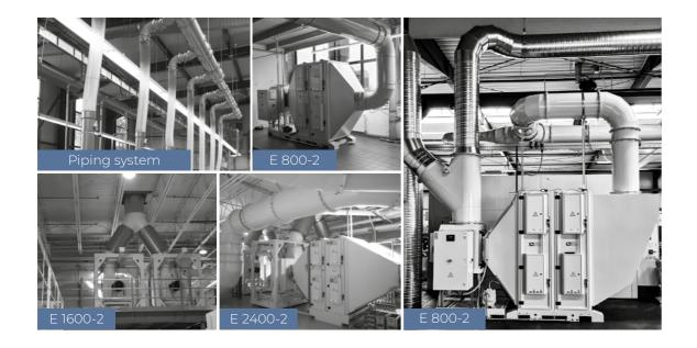
Electrostatic filtration systems for oil and emulsion mist are the ideal solution to sustainable production in industry and trade. The prefilters and main filters are completely washable and therefore reusable. As extremely flow-optimized solutions, the electrostatic filters for coolant mist stand for a long service life, as well as long-running and consistently high performance. All applicable industrial and authority requirements are fulfilled without compromise.
